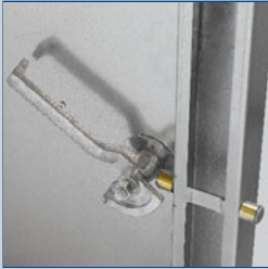
Double lever locking device – interior lever
