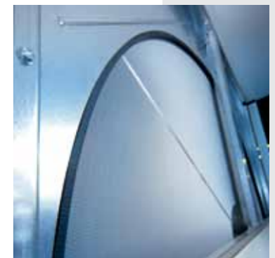
Rotary heat exchanger
